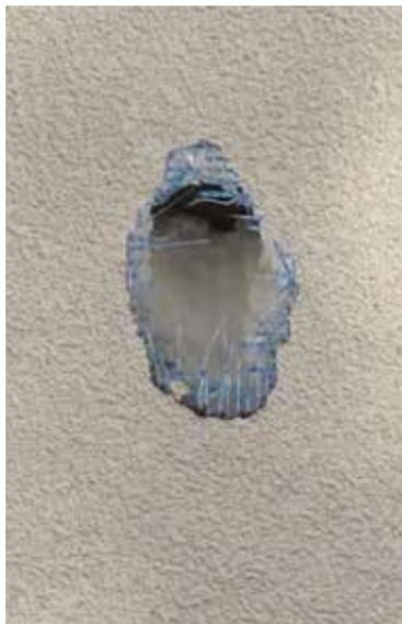
Examples of damage to buildings caused by parakeets
