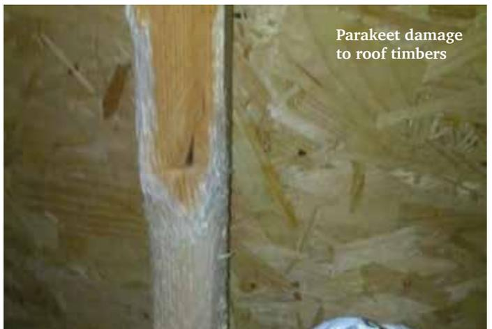
Parakeet damage to roof timbers
